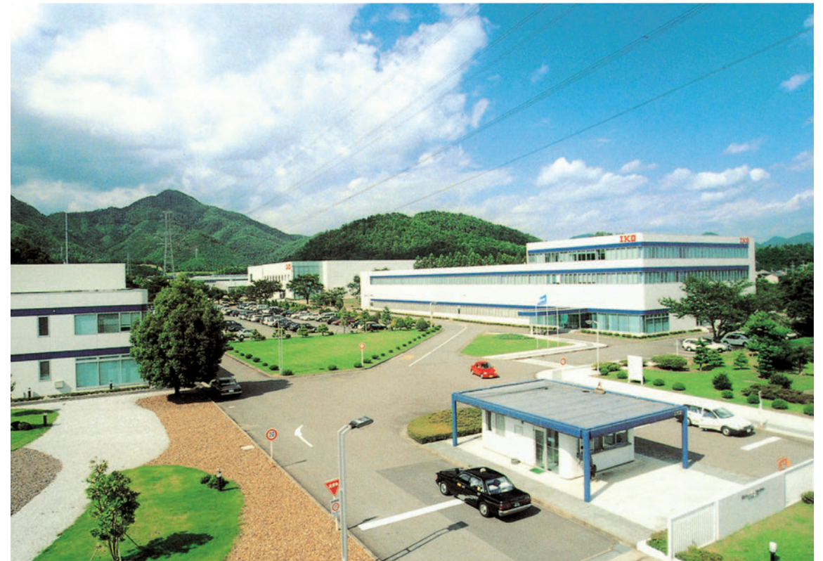
Gifu factory main entrance
